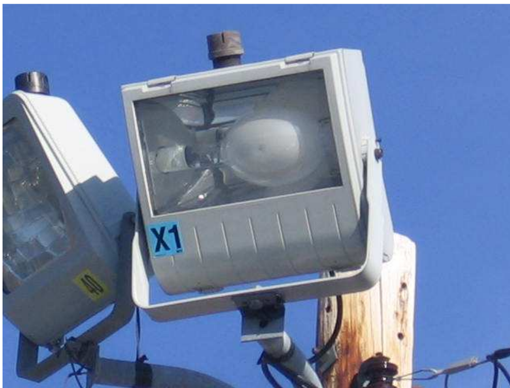
High-power, high-pressure, unshielded sodium floodlight.
