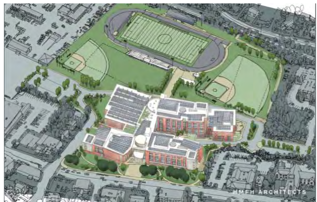
Figure g: Aerial Site Overview
