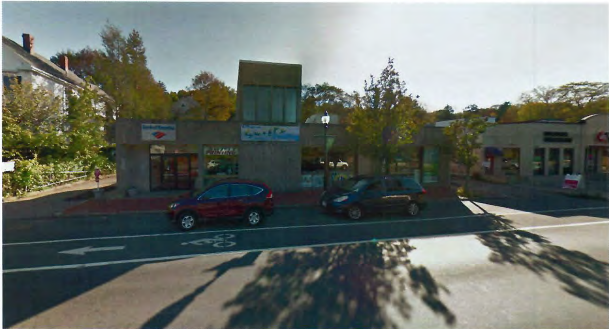
Figure 1 – 1386 Massachusetts Avenue, Arlington, MA © Google Image Capture
