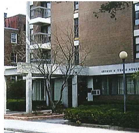
O'Shea house, Brookline Housing Authority property, 100 units of affordable housing, VRF heat pumps.
