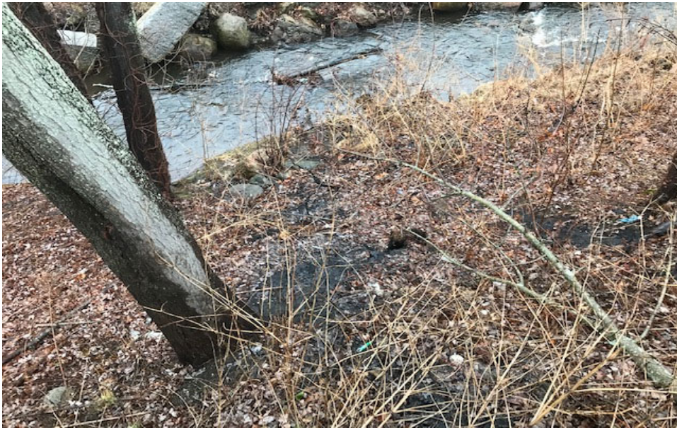
Figure 7: Northern view of bank behind grease trap.
