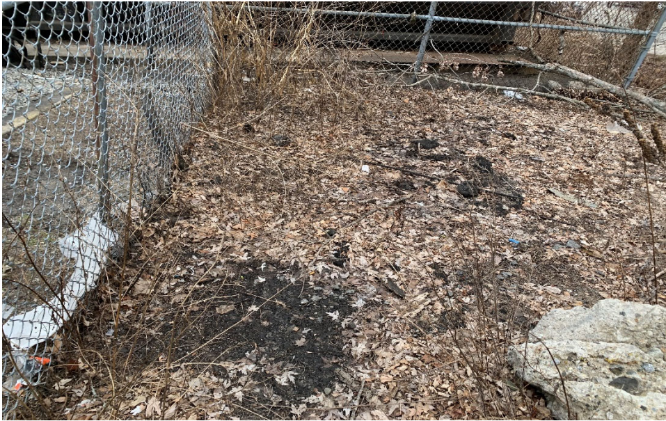
Figure 5: Western view of top of bank behind grease trap.
