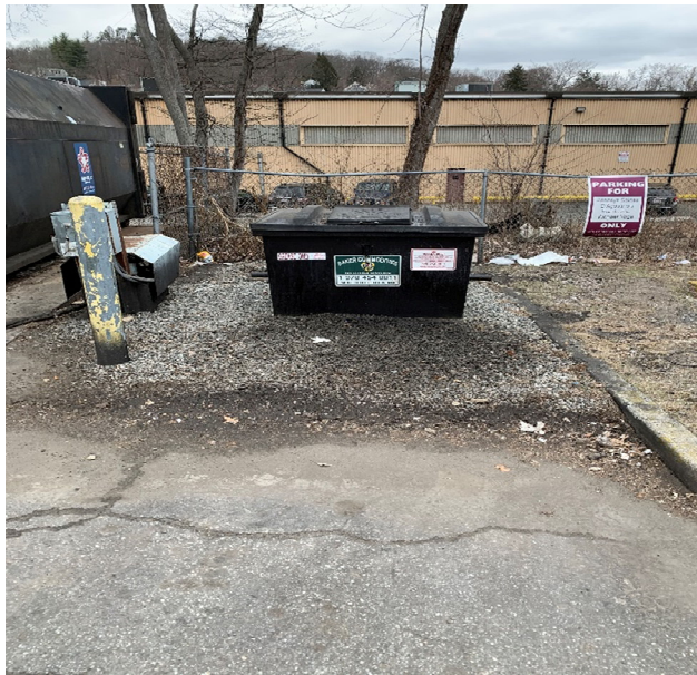
Figure 3: Northern view of front of grease trap.
