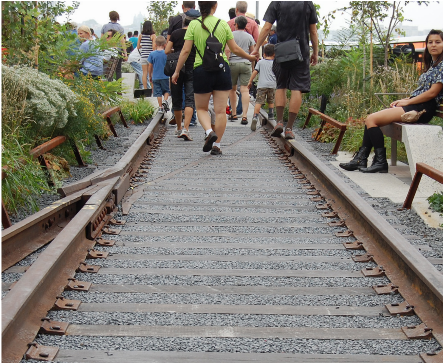
Resin-bound aggregate paving between existing tracks.
