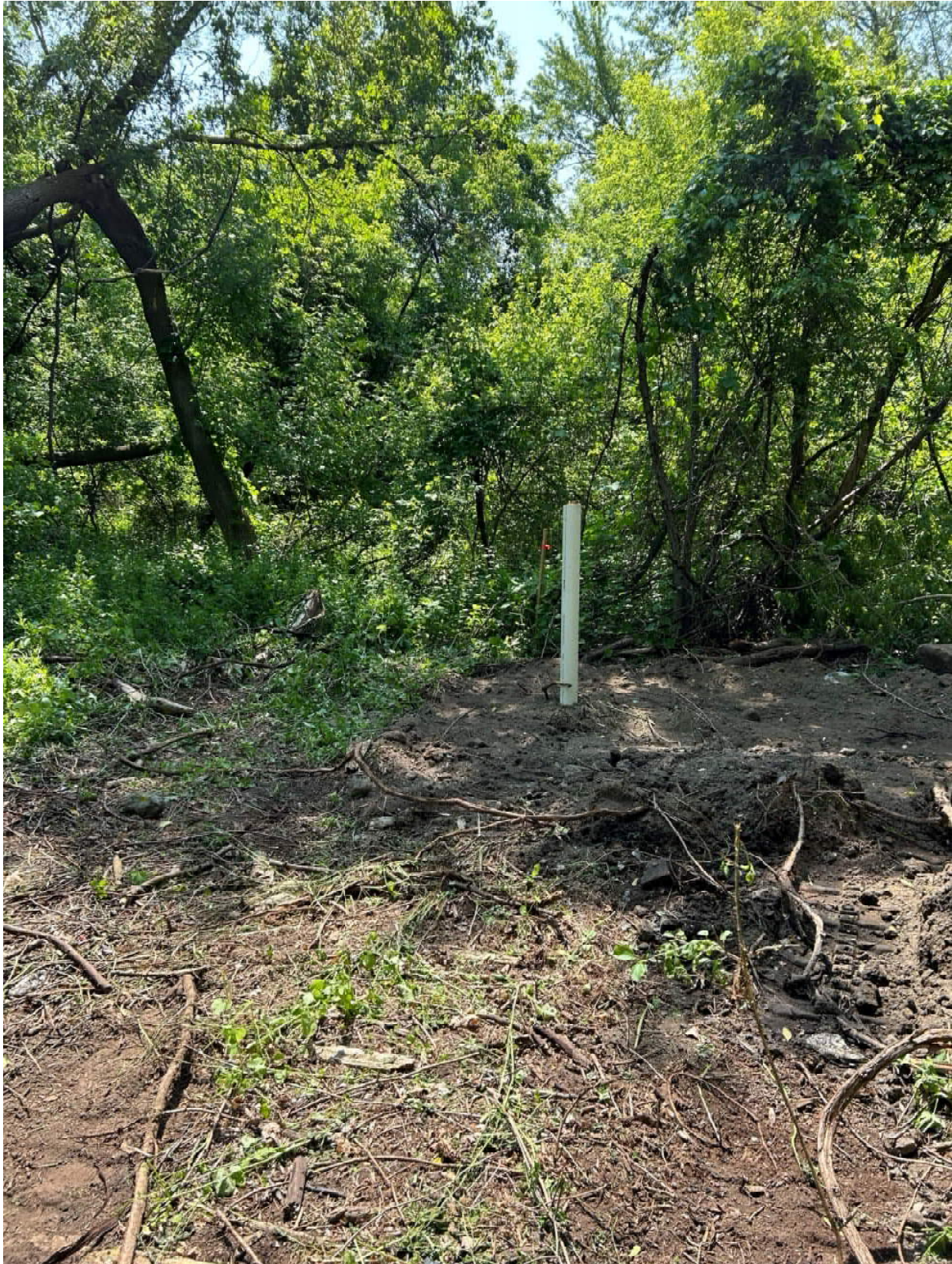
Completed monitoring well at TP-7
