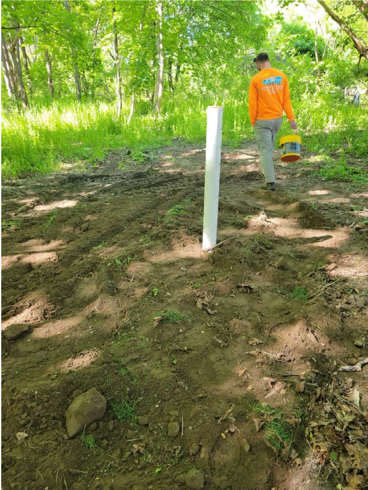
Completed monitoring well at TP-1
