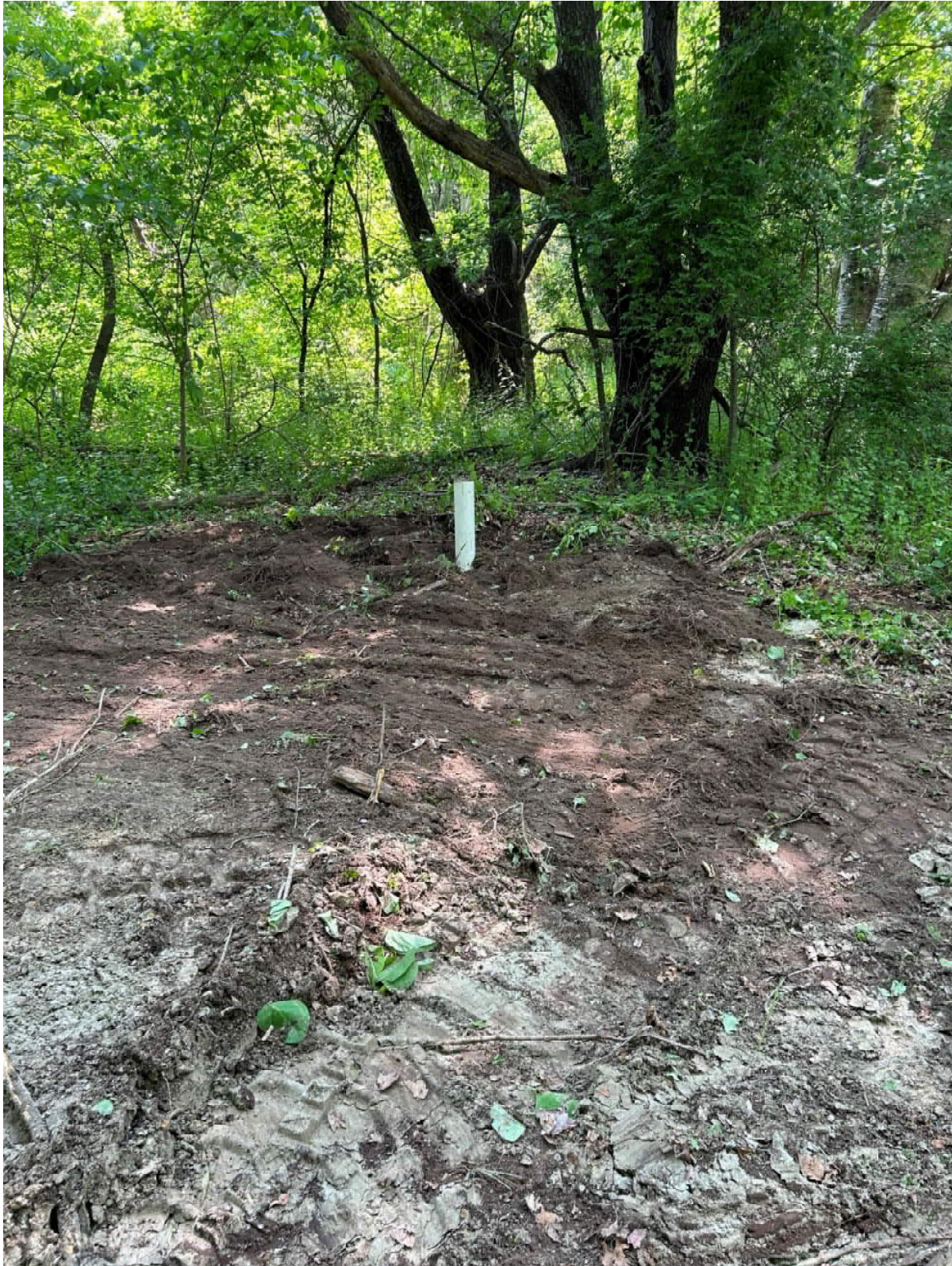
Completed monitoring well at TP-6
