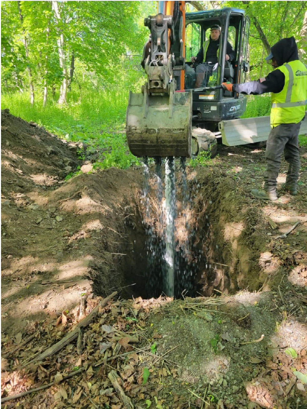
Installation of monitoring well at TP-1
