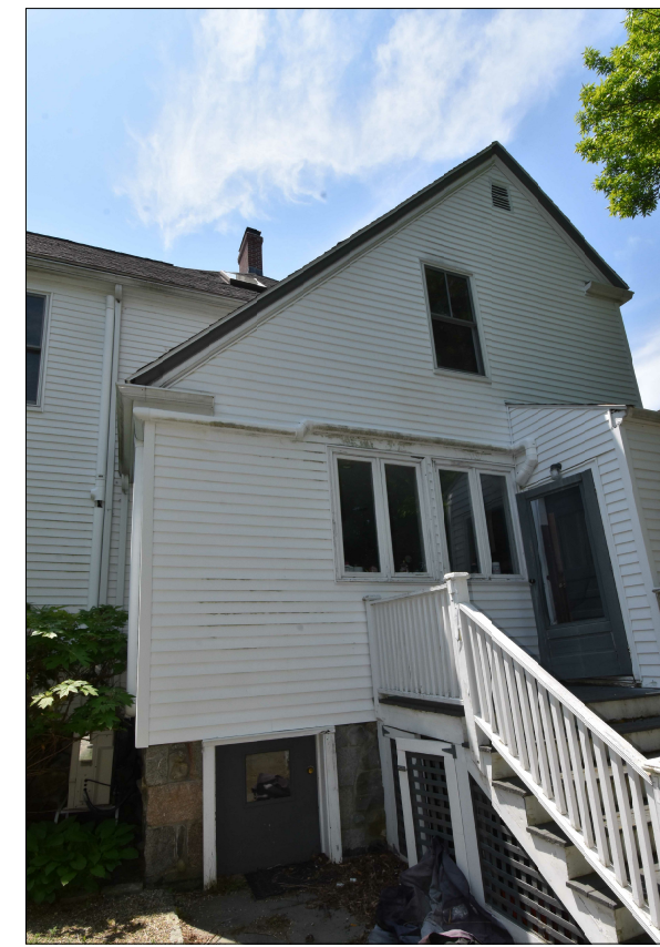
Existing Rear Facade
