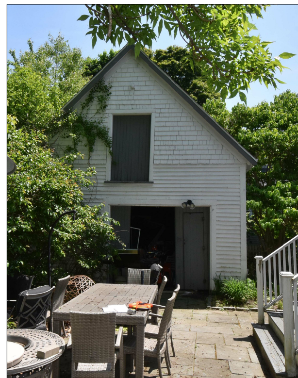
Existing Barn Entry Facade
