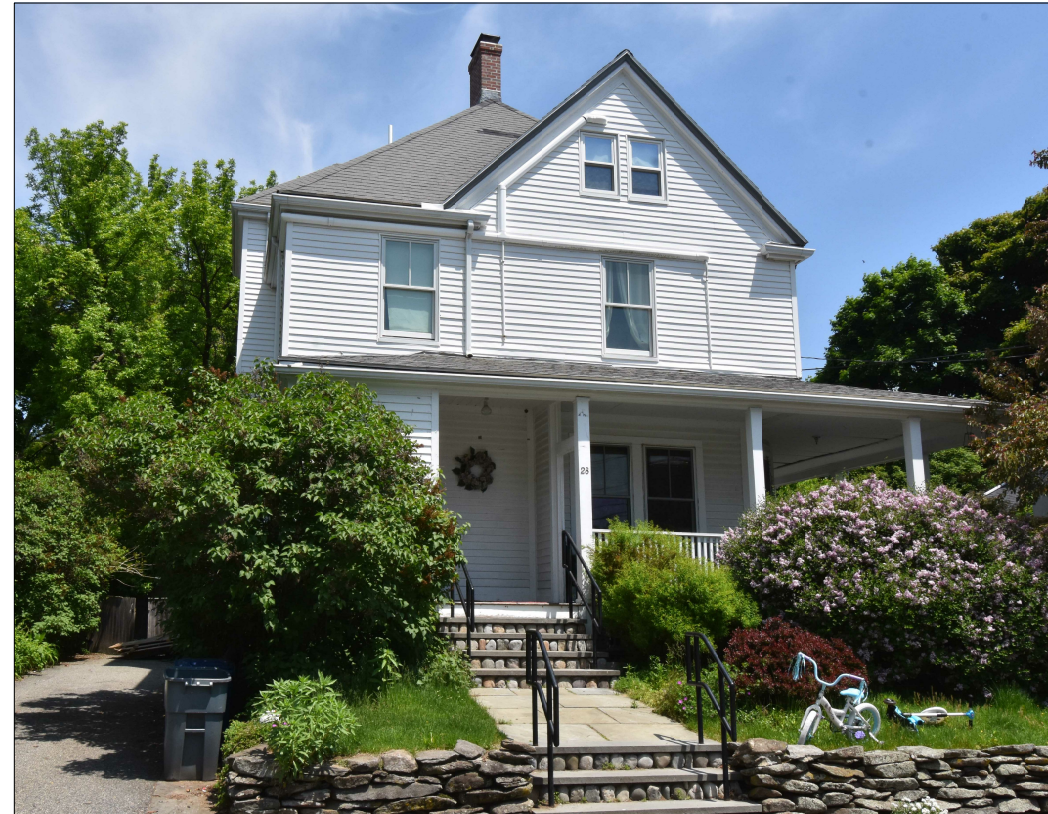
Existing Street Facade
