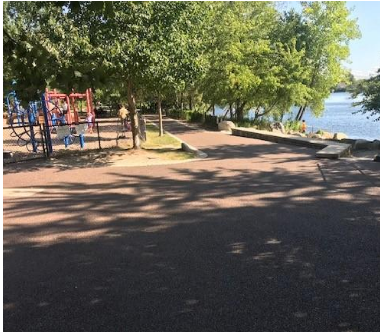
The Spy Pond Project included resurfacing the pathway with an ADA accessible porous pavement.
