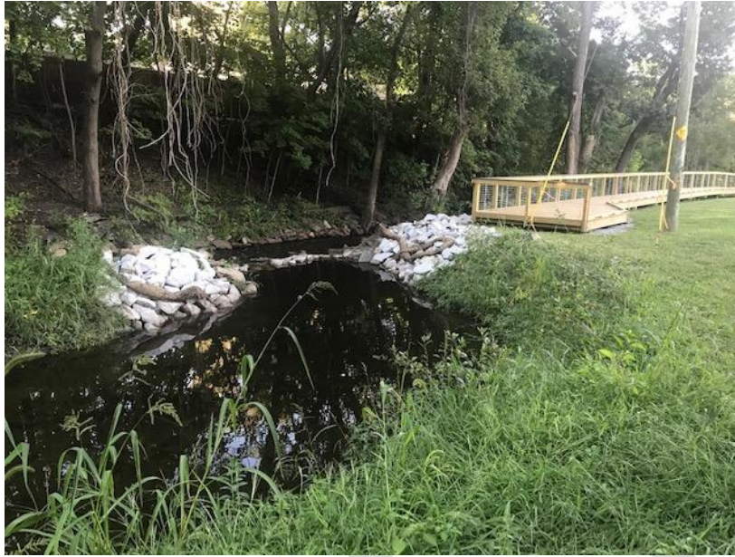
The flood storage area slows floodwaters downstream of Wellington Park.
