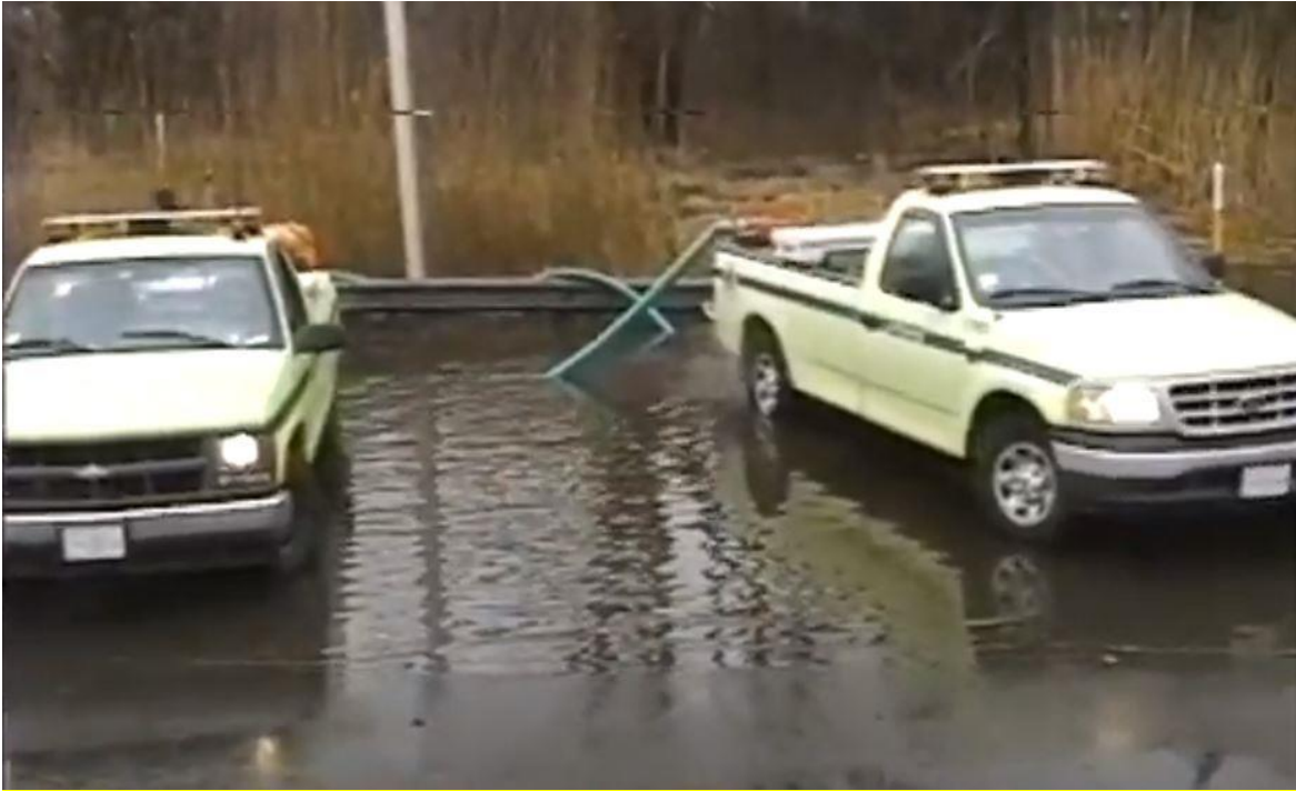
Figure 5. DPW pumping from Route 2 to into Mugar site wetlands during 2001 storm
