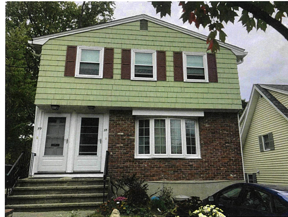
EXISTING STREET VIEW
