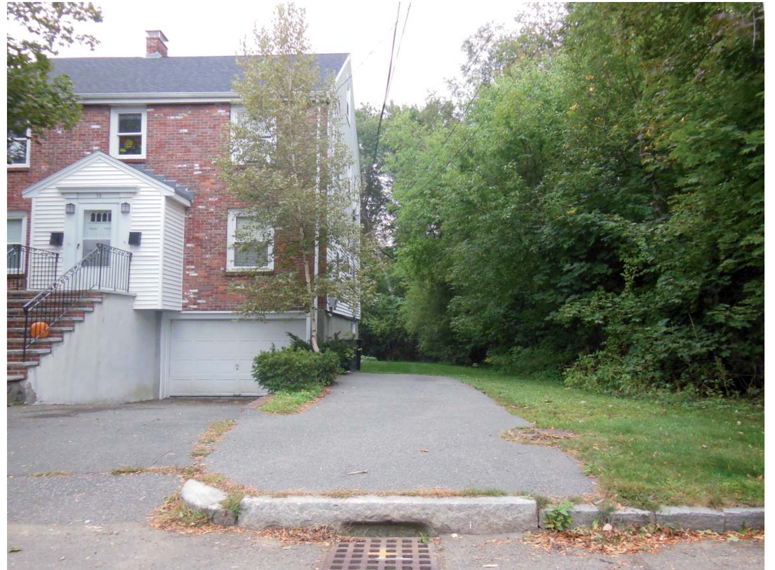
Dorothy Road home adjacent to site.
