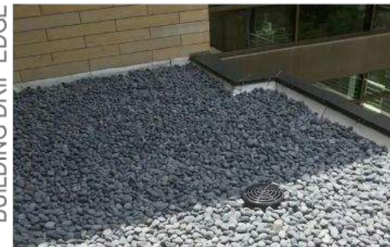
Drip edge between building and planters (8" offset)
