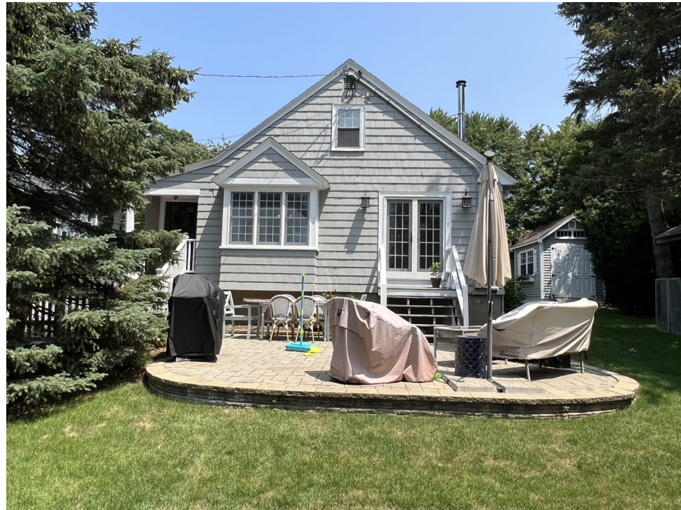
Right Side Facade
