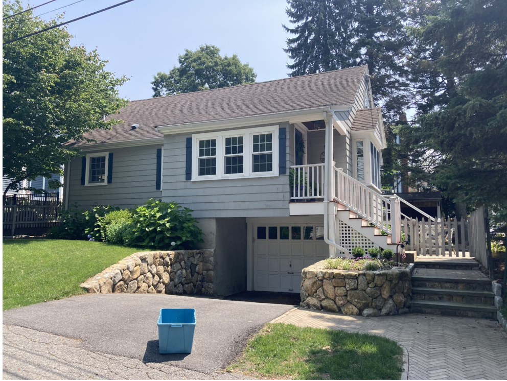
Street Facade - Front
