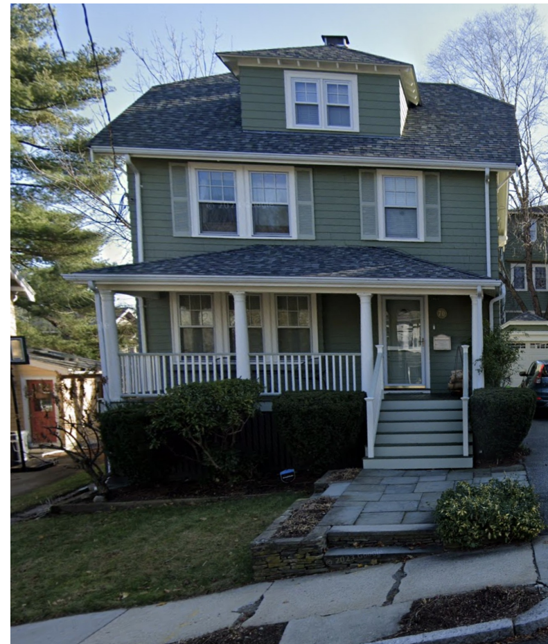
70 ROBBINS ROAD, EXISTING
