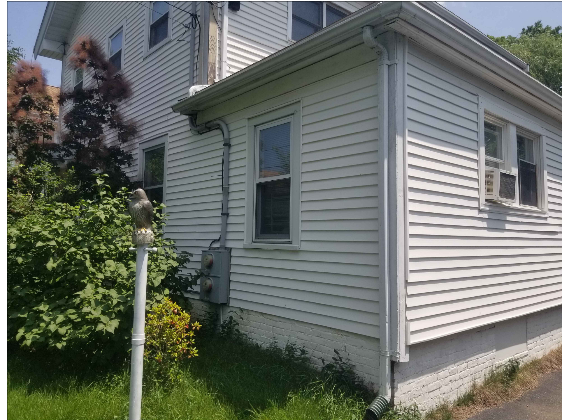
IMAGE 5 FRONT RIGHT CORNER
