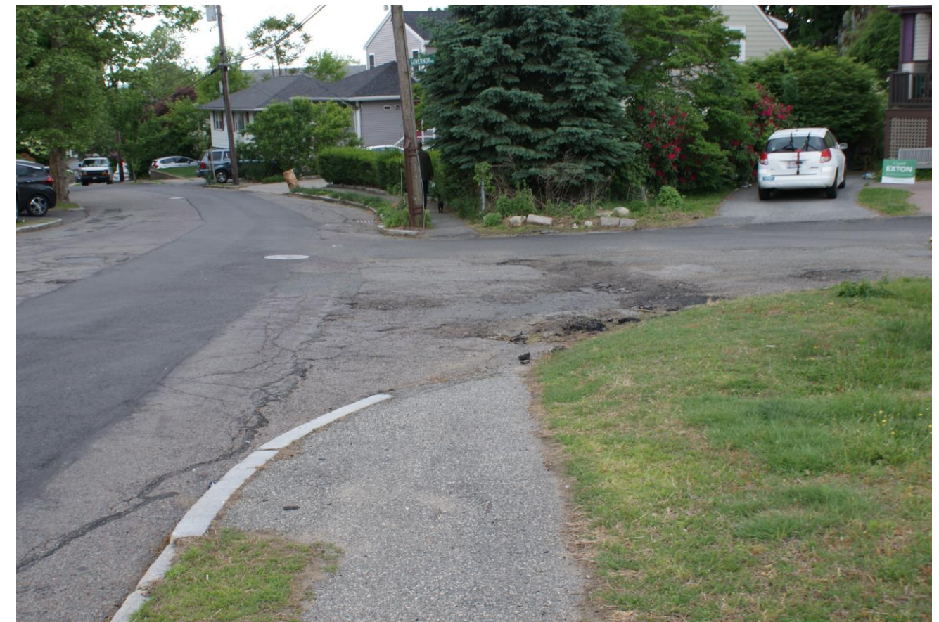
Missing crosswalks across side streets.
