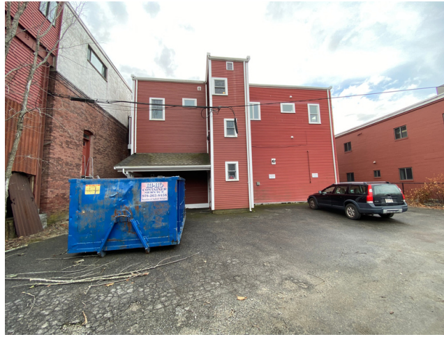
12 North Side (Back) View
