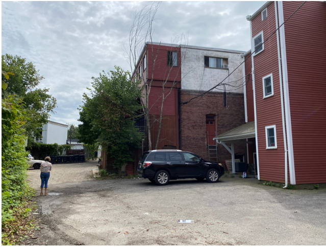
11 Rear Lot View looking East.
