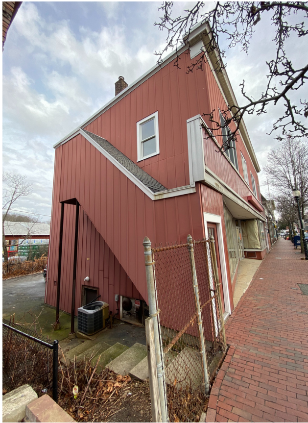
1 West Side at South corner.
