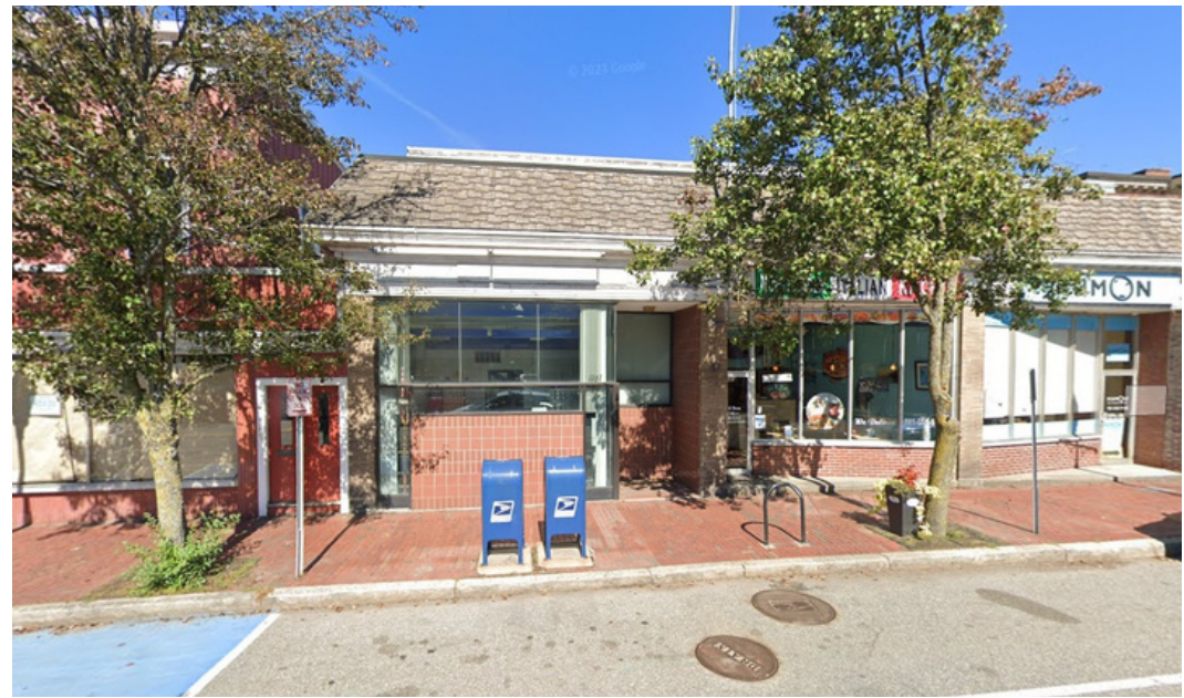
4 1347 Mass Ave. (Adjacent Building. )
