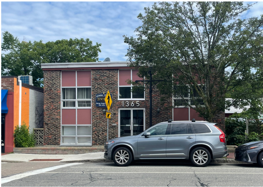
3 1365 Mass Ave. (Adjacent Building)
