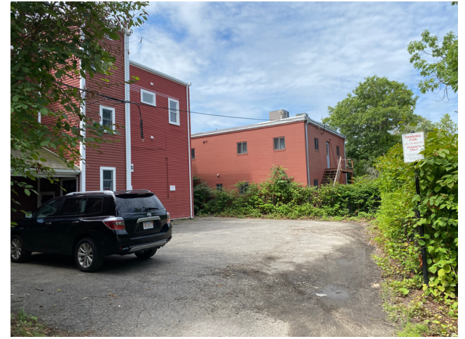
13 Rear Lot Looking to the West.
