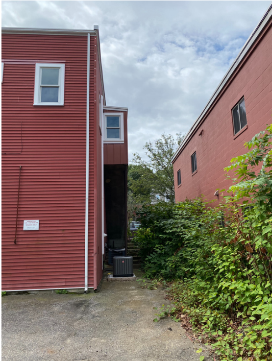
14 Alley on West Side looking South.
