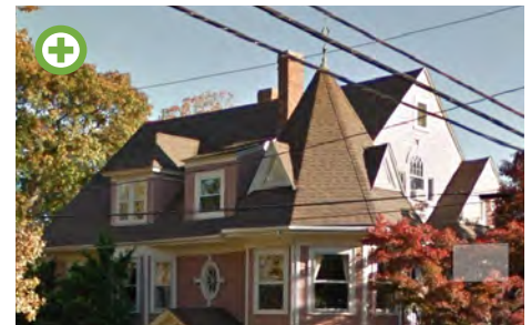
Gable roof with corner turret and dormers. (Source: Google Streetview)
