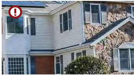
Multiple materials are used, but it is obvious that the stone material is merely "stuck on." Source: Google Streetview.
