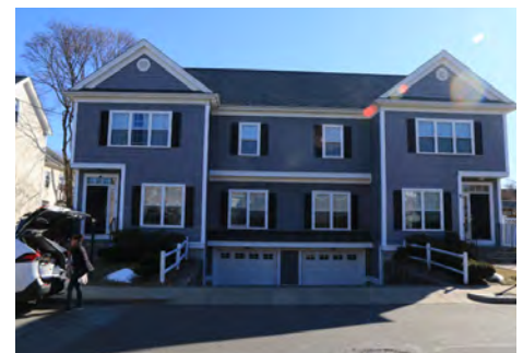
Examples of “Park-Unders” built before the new slope regulations were put into place.
