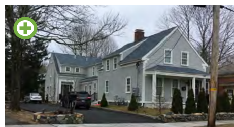
Consider pairing a larger unit with a smaller unit, either to the side or rear, to break the massing apart. Source: DRWG.
