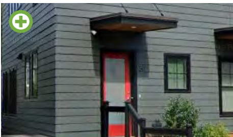
Contemporary entryway. Source: Google Streetview.
