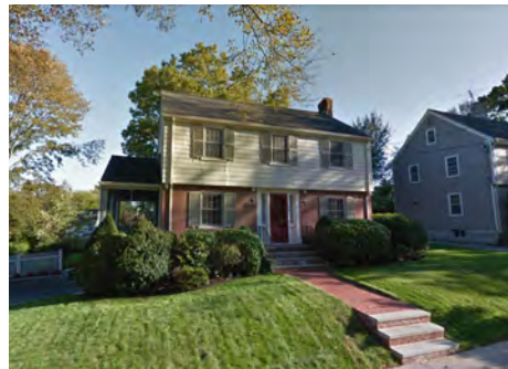
Example of a 'Garrison' Colonial built in the mid-20th century. Source: Google Streetview.
