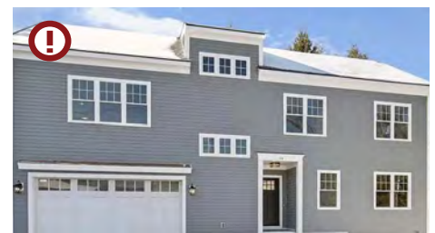
Windows are not ordered or aligned in a logical fashion. Source: Google Streetview.
