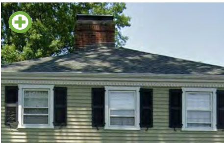
Window trim meets the bottom of the roof without a big gap. (Source: Google Streetview)
