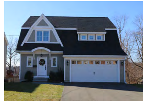
Example of a New Traditional colonial-styled house built in the 2010s.
