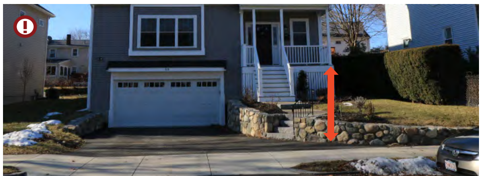
The foundation height of this house greatly exceeds the house's neighbors due to the attached garage. Source: Harriman.
