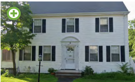
Windows do not necessarily align vertically but are ordered and symmetric. Source: Google Streetview.
