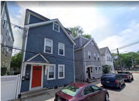
Oversized shed dormers on gable roof effectively create three-story houses; South Boston, MA. Source: Google Streetview.
