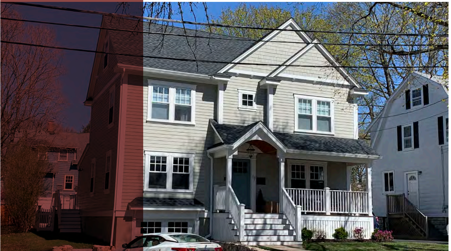
New construction in Arlington Heights.
