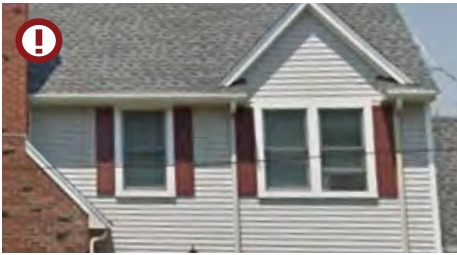
Shutters are purely decorative and do not appear 'functional.' Source: Google Streetview.
