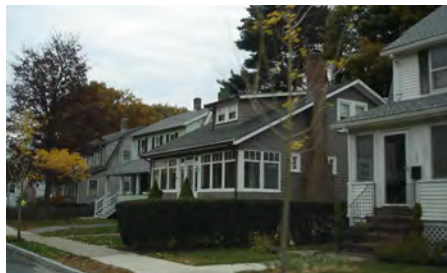
Example of a Bungalow-style house. Source: Google Streetview.
