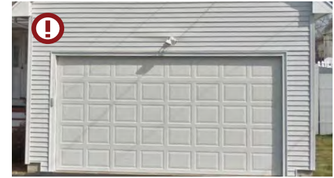
Plain garage doors are fine in the rear but not in a prominent front area. Source: Google Streetview.
