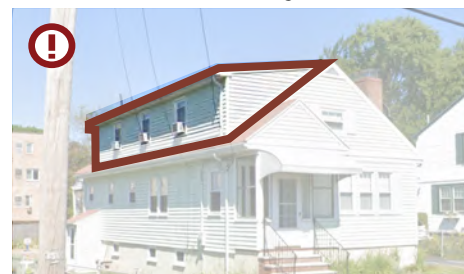
While the height is not excessive, the dormer is too large relative to the house. Source: Google Streetview.
