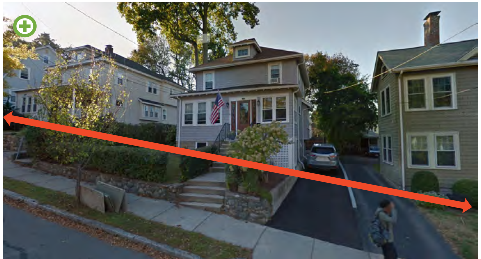
Use a consistent foundation height that matches the pattern of other houses on the street. Source: Google Streetview.
