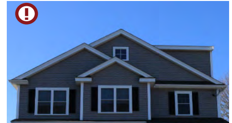
Complex combination of gable roofs and low-pitched roof with high eaves makes house appear taller. (Source: Harriman)
