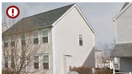
Blank side face with no windows. Source: Google Streetview.
