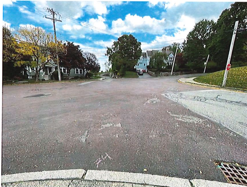
Looking south-east from the intersection of Endicott and Gloucester
