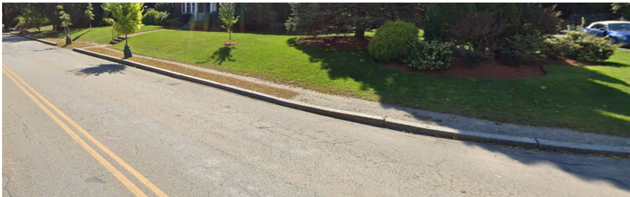
Figure 2: White Edge line along Gray St is no longer visible from some angles
