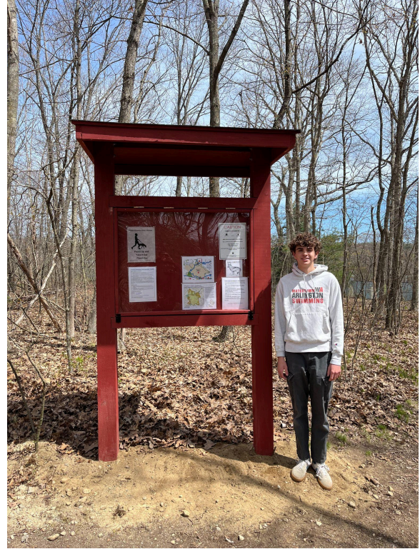
Picture of the finished product of the kiosk the day after the project execution. This was once the concrete had set and we removed the braces that we used to ensure the kiosk wouldn’t shift around while the concrete was drying.
