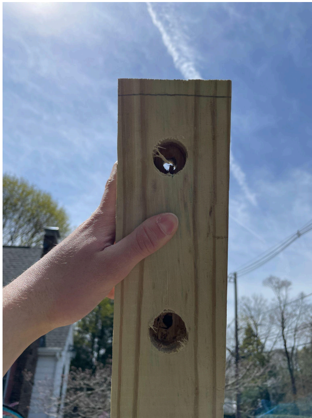
Drilled Pilot holes in one of the 4x4 posts to secure the "Arlington's Great Meadows" sign to the posts with carriage bolts, nuts, and washers.
