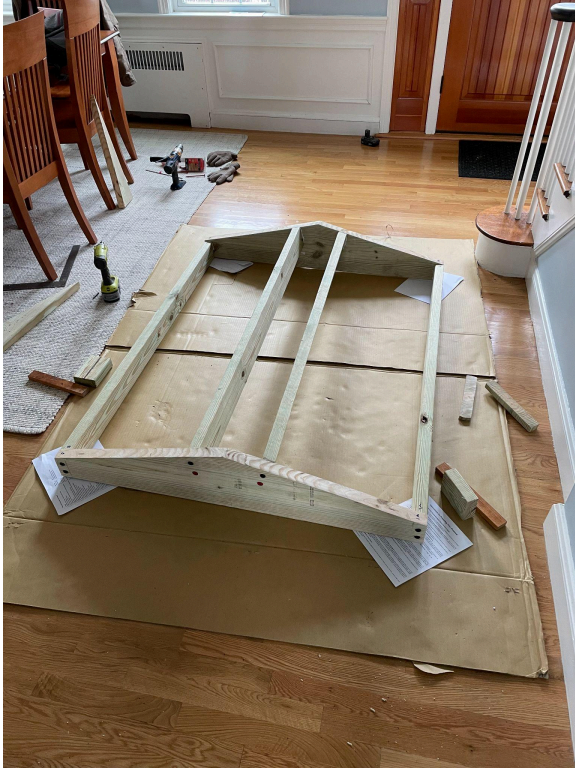
Roof skeleton with 2x4 cross supports attached.
