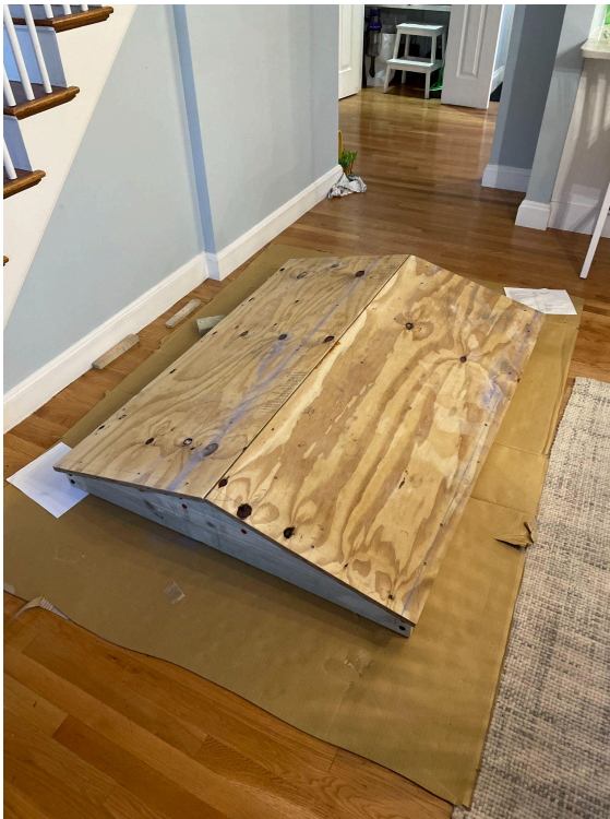
Finished roof structure with plywood attached.
