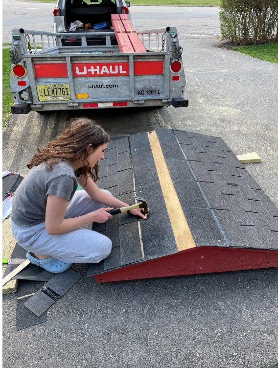
Nailing down the shingles onto the roof.
