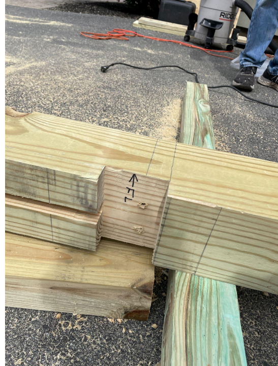
"FL" written on the 6x6 post to indicate that where the arrow is pointing is the front left side of the kiosk.
