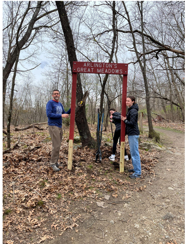
Preparing to put the posts of the “Arlington’s Great Meadows” sign into the post holes.
