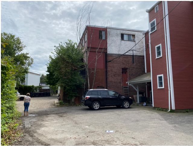
11 Rear Lot View looking East.
